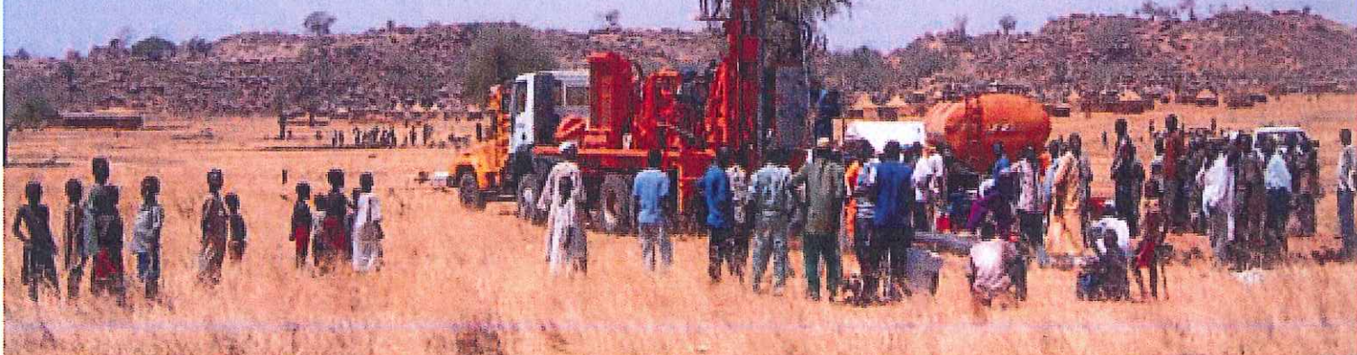
Watertec 10 water well project in Sudan
